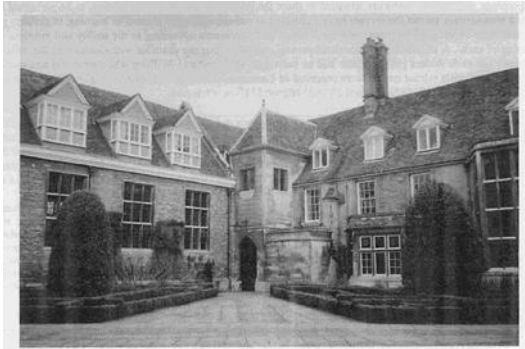
Figure 11. New Court, Emmanuel College, Cambridge in April 2006. The old chapel is on the left and the hall on the right.
