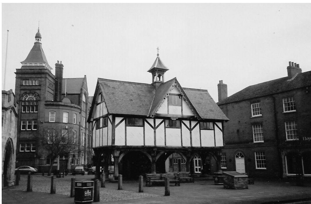
Figure 25. The former Grammar School, Market Harborough, Leicestershire in March 2004. The wooden strips on the outside of the upper part are not part of the original structure and the bell-turret was added in 1868.
