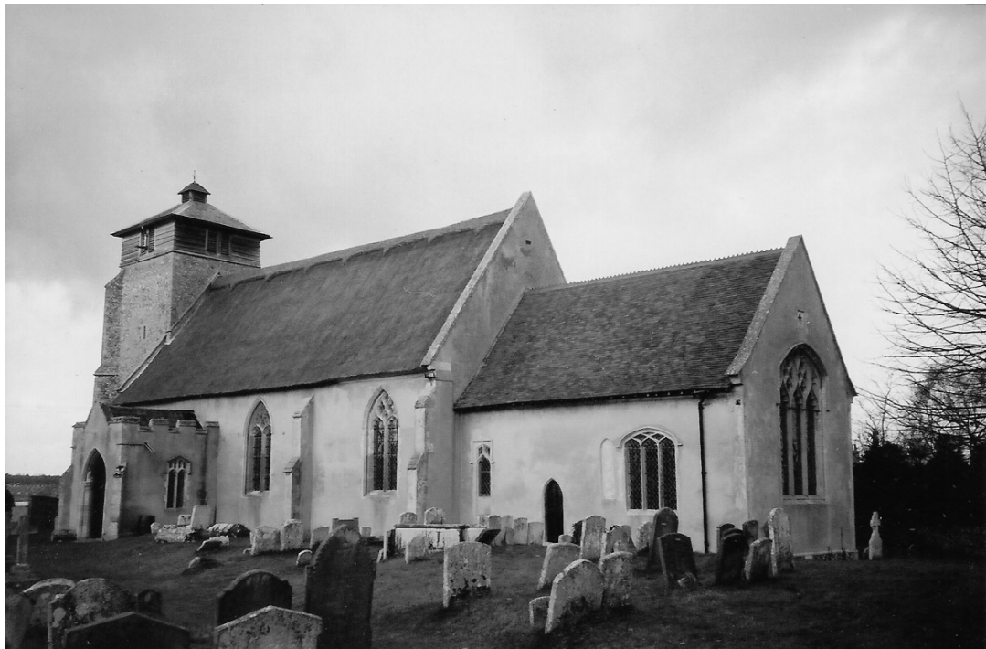
Figure 29. The church of St Peter, Great Livermere, Suffolk in March 2006. The short top to the tower was built after the previous turret fell off in a storm in the 1870s.
